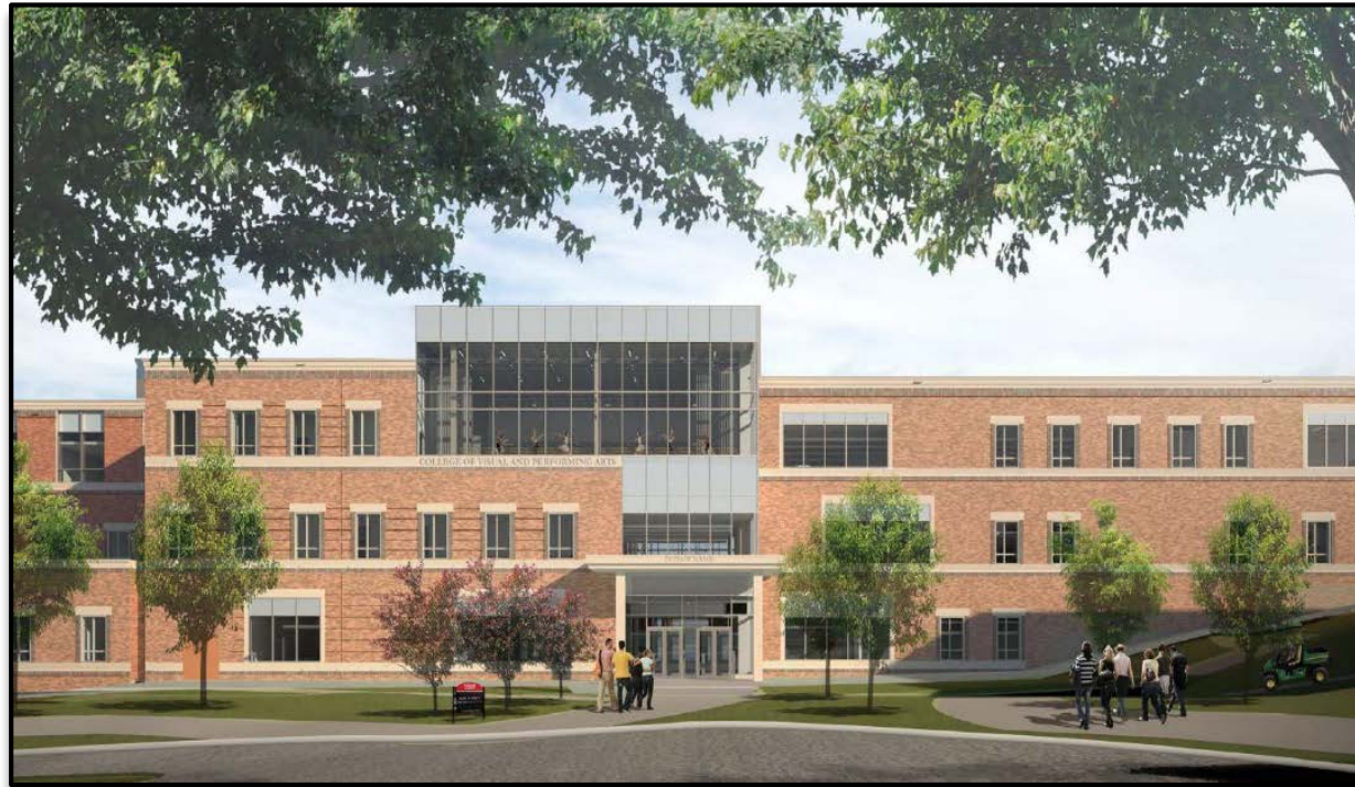
View from Parking Lot A
